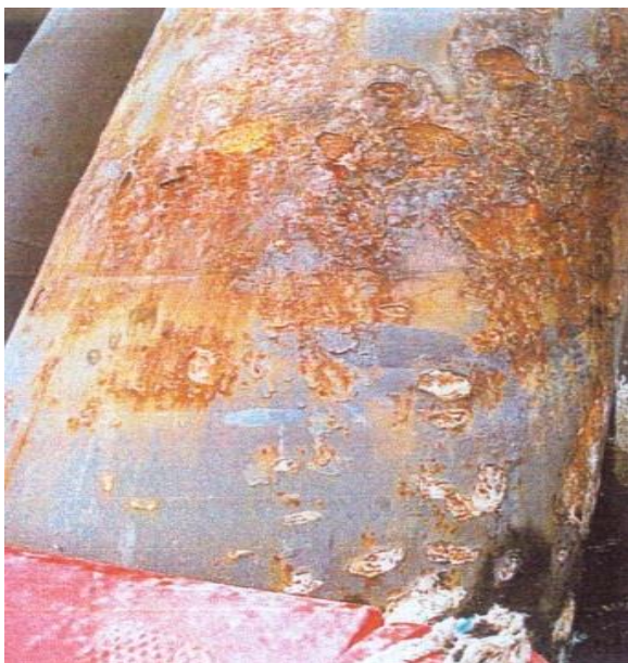
Fig. 62: Coating damage in tidal zone [27].
